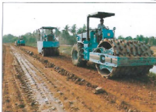
Cambodia: Compaction of the road surface. The road construction methods using Con-Aid in this area are the same as those used in South Africa and, as in South Africa, provide a high-quality, low-cost road by making use of in-situ materials, as well as materials normally considered unsuitable for road construction.
