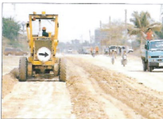
A Con-Aid road in the process of construction in a city in Thailand. Due to the high volume of traffic it is impossible to close the road and work has to be done without interfering with the flow of vehicles. The use of Con-Aid minimises this problem.
